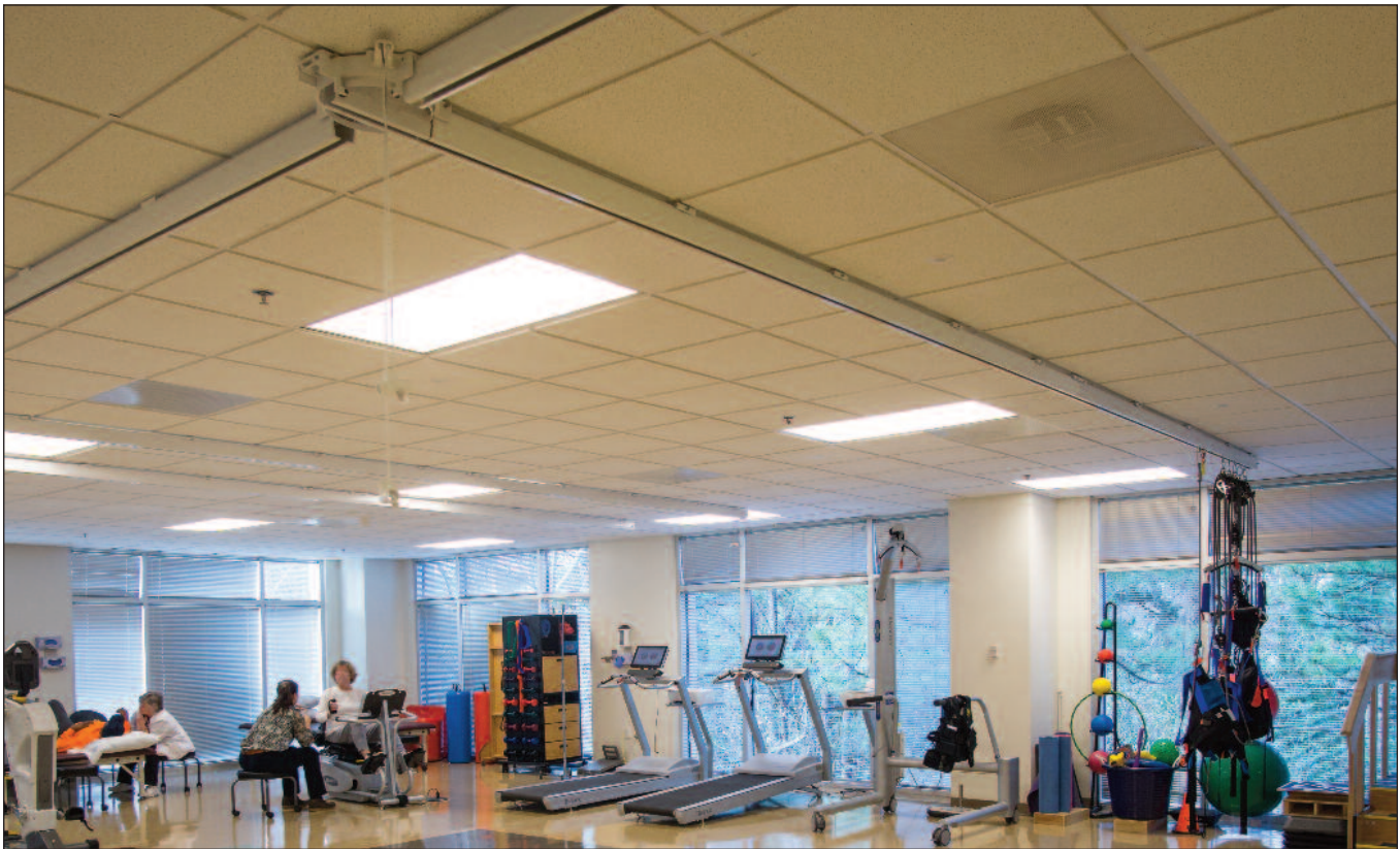
The Emory outpatient neurorehabilitation clinic focuses heavily on helping patients with Parkinson’s disease recover their ability to ambulate safely in the community – and thus, has installed one of the world’s most extensive overhead track systems, 220 feet of Biodex FreeStep SAS that enables patients to practice walking and performing occupational therapy in a kitchen or laundry area without risk of a fall.
